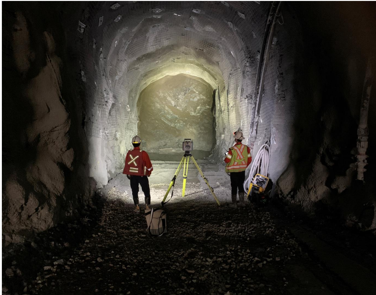
Red Chris Exploration decline has advanced 319 metres as at 29 September 2021
